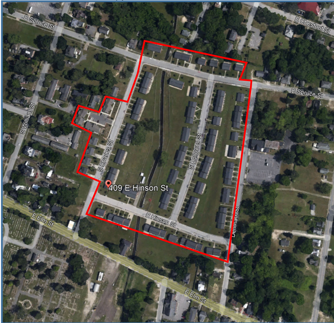
Figure 15. Recommended NRHP Boundary for Elmwood Terrace Apartments outlined in red.
