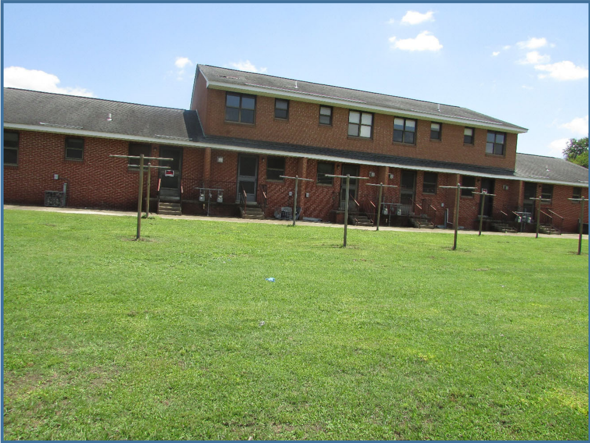
Figure 5. Elmwood Terrace Apartments, building D-35 rear elevation, view to east.
