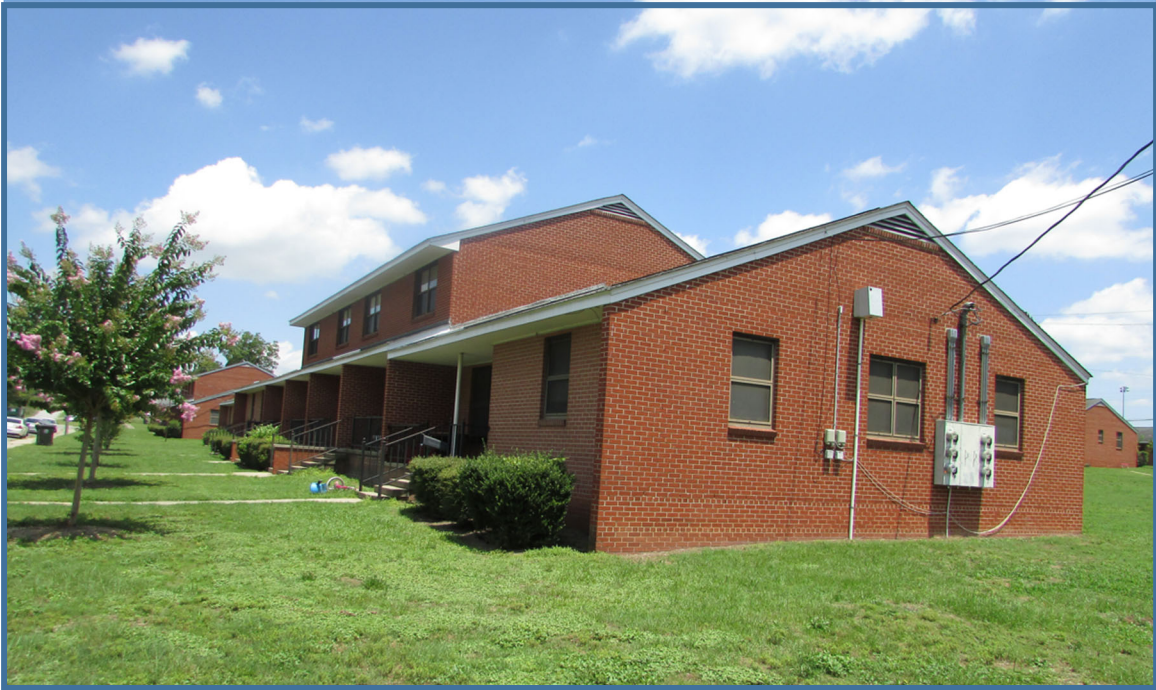
Figure 12. Woodcrest Apartment, Goldsboro, North Carolina.
