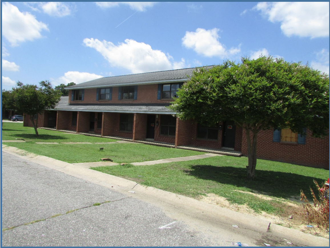
Figure 4 Elmwood Terrace Apartments, building facade D-23, view to the south.
