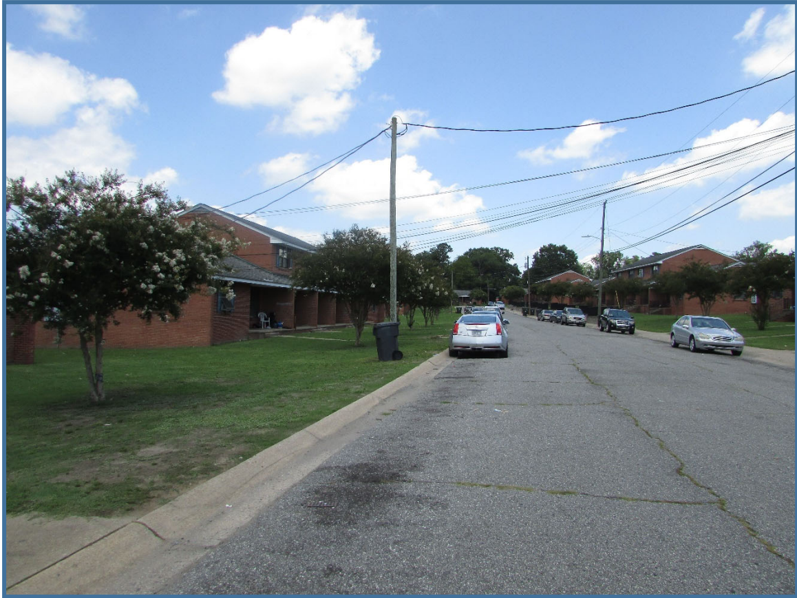
Figure 8. Elmwood Terrace Apartments, Smith Street, view to the north.
