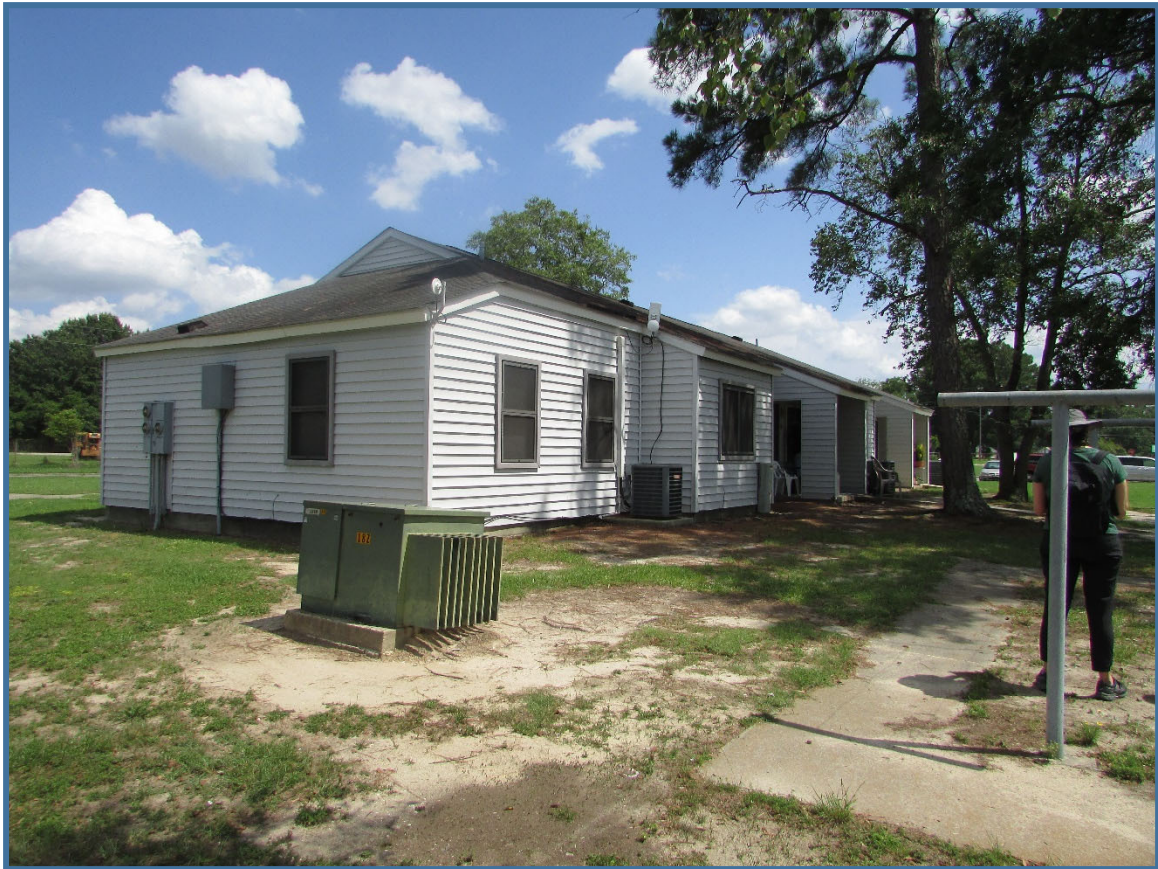
Figure 5. West Haven Apartments, 133-137 Dupont Circle, rear elevation, view to southeast.
