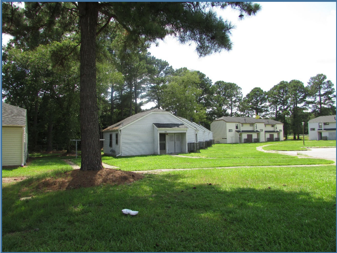
Figure 10. West Haven Apartments, 829-835 W. Oak Street, view to the west.
