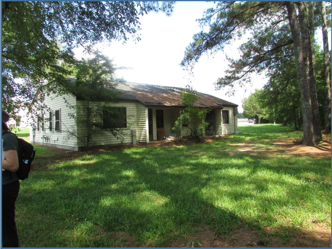
Figure 15. West Haven Apartments, 919 W. Oak Street, view to the south.
