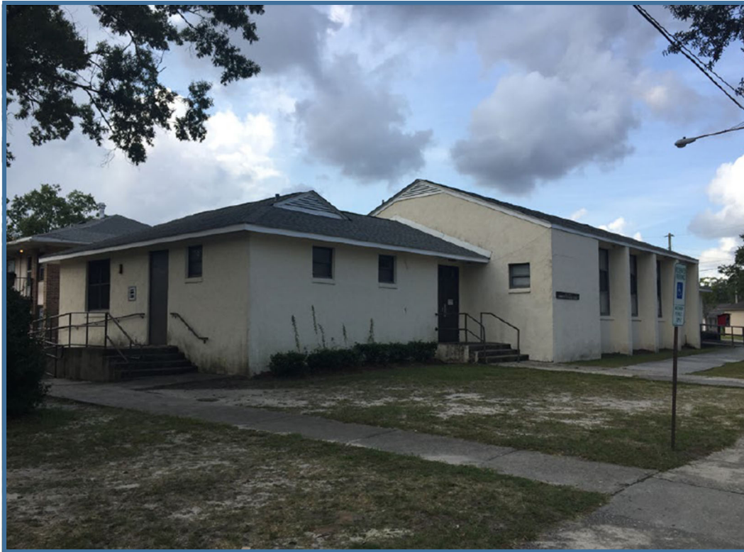
Figure 29. Hillcrest and Hillcrest Annex Public Housing Complex.
