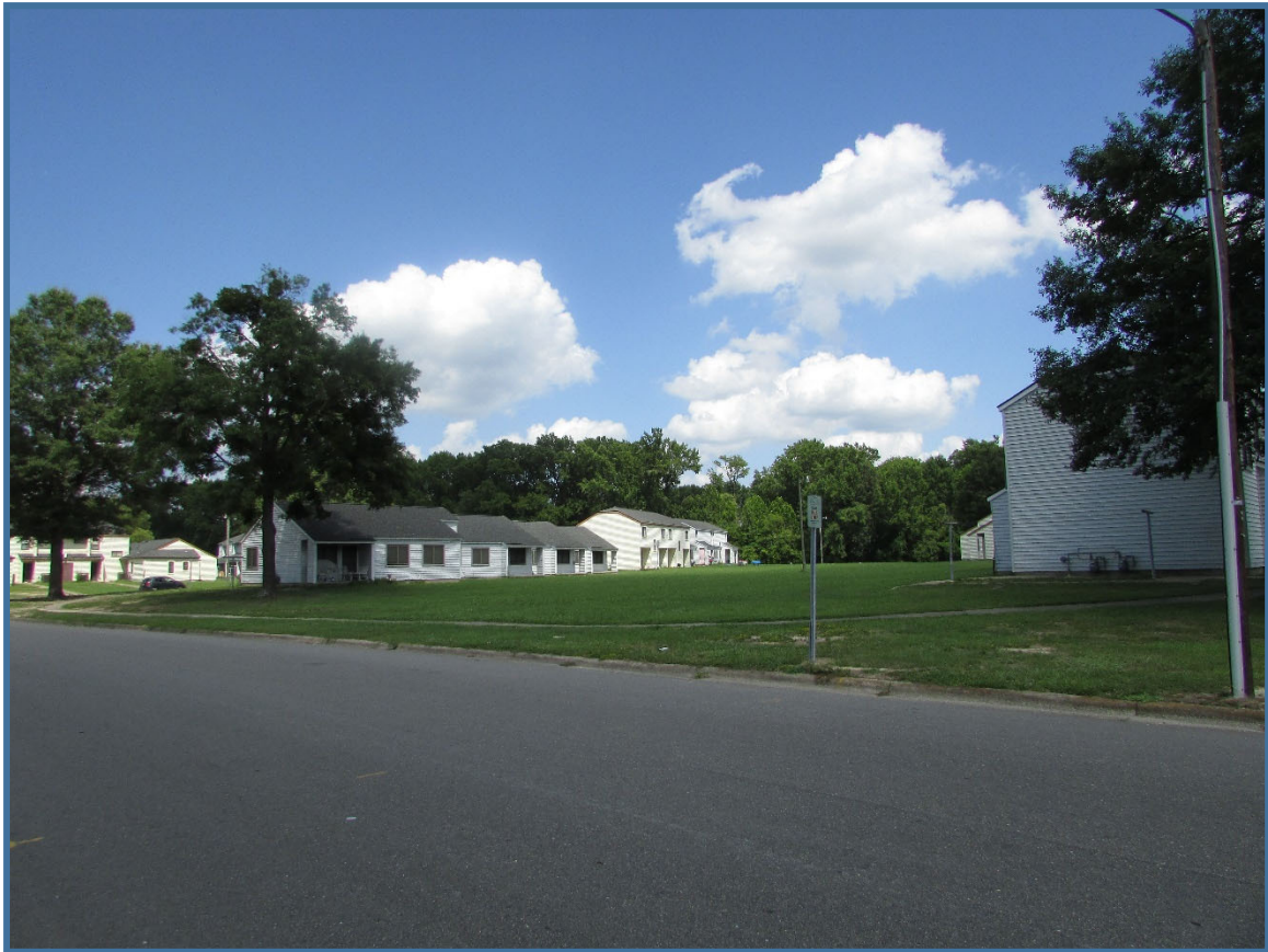
Figure 16. West Haven Apartments, Vanderbilt Circle, view to the northeast.
