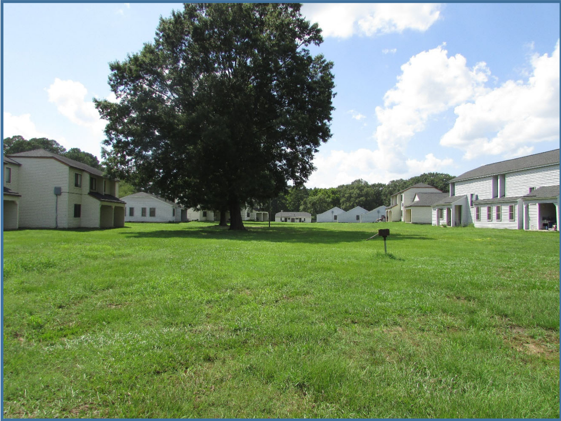
Figure 9. West Haven Apartments, common area, view to the west.
