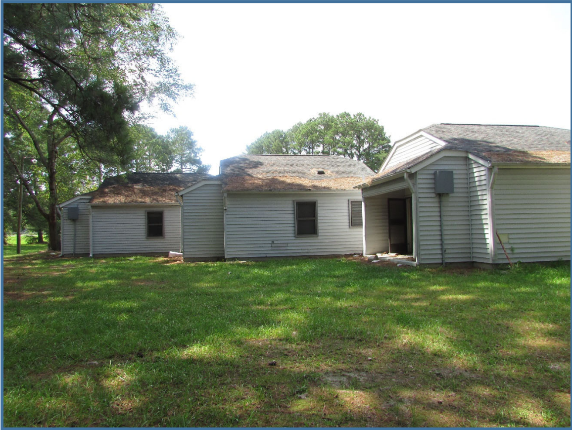
Figure 14. West Haven Apartments, 911-917 W. Oak Street, view to the south.
