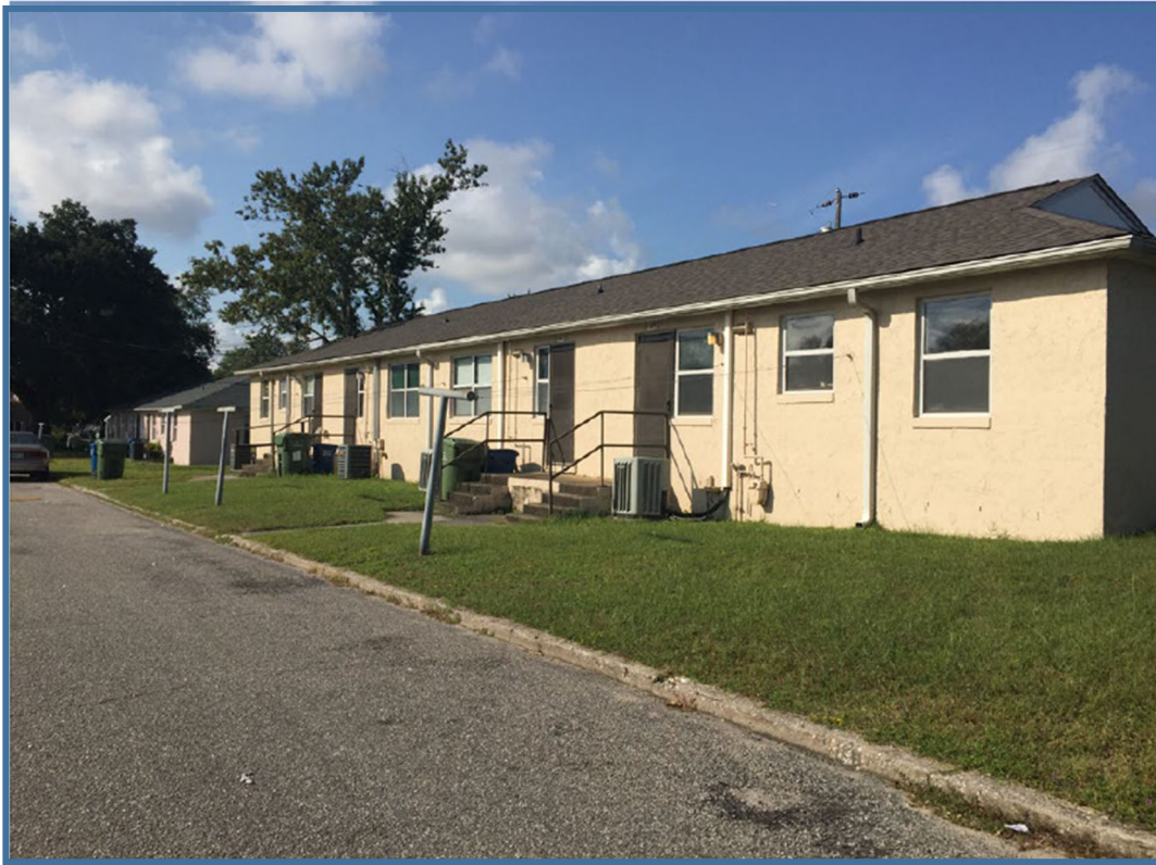
Figure 28. Hillcrest and Hillcrest Annex Public Housing Complex.
